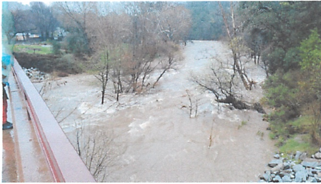
Downstream from Bridge
