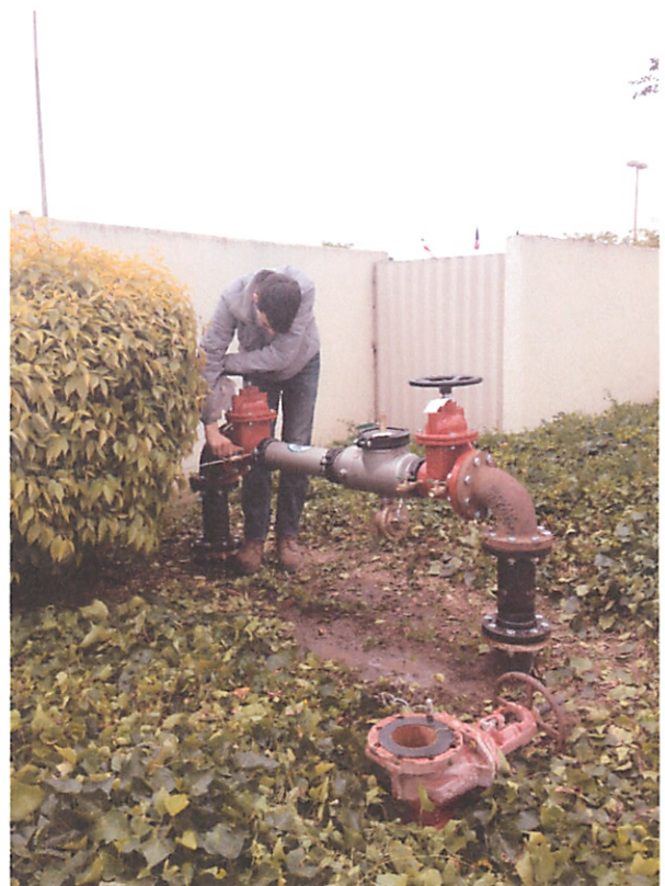
Eli finishing up the new Backflow Valve for Fox Shox in Watsonville - June 2016
