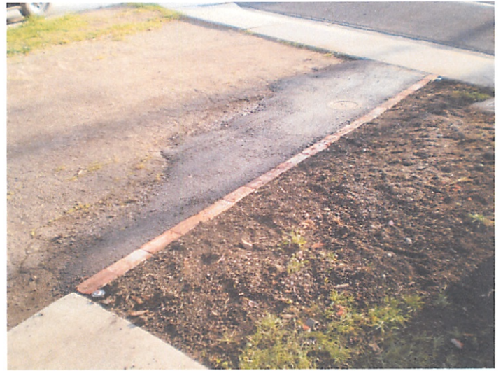
Brick Lawn Edging and new Driveway Asphalt at end of day
