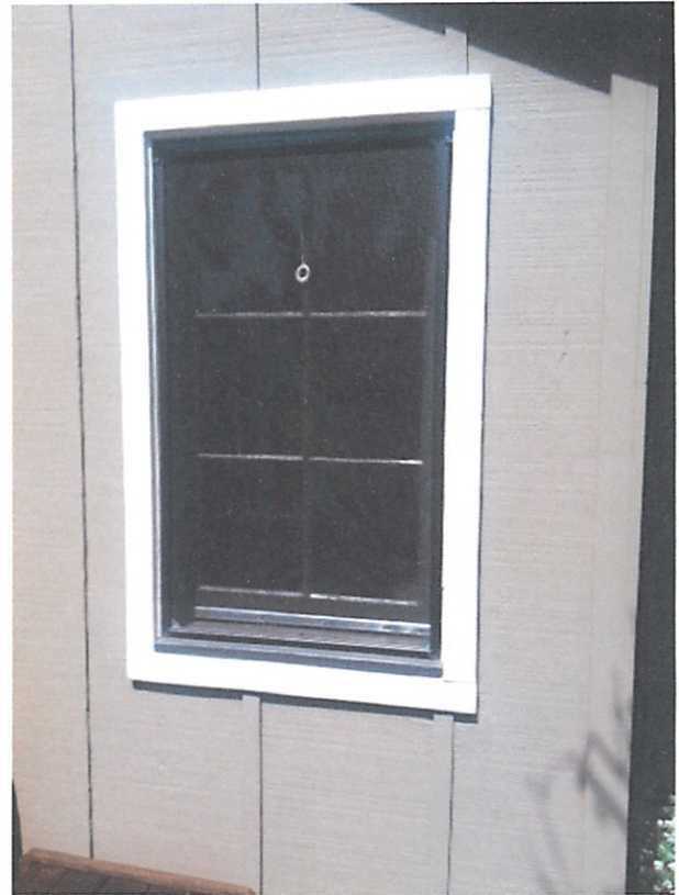
One of the original front windows of cabin.
