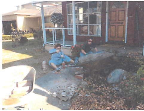
Robin & Nancy chipping mortar off of old bricks
