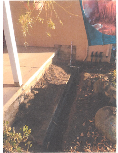
Trench for footing of new planter and sprinkler system valves
