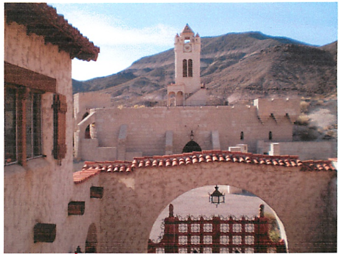
Unfinished Wing from Bridge over Stableyard
