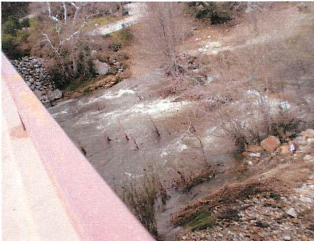
River rushing under bridge Bridge rail lower left
