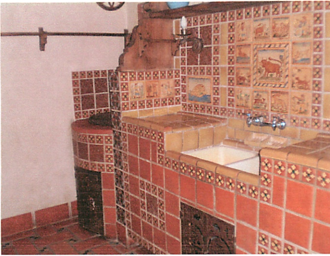
Cold and Solar Hot Water Sink
