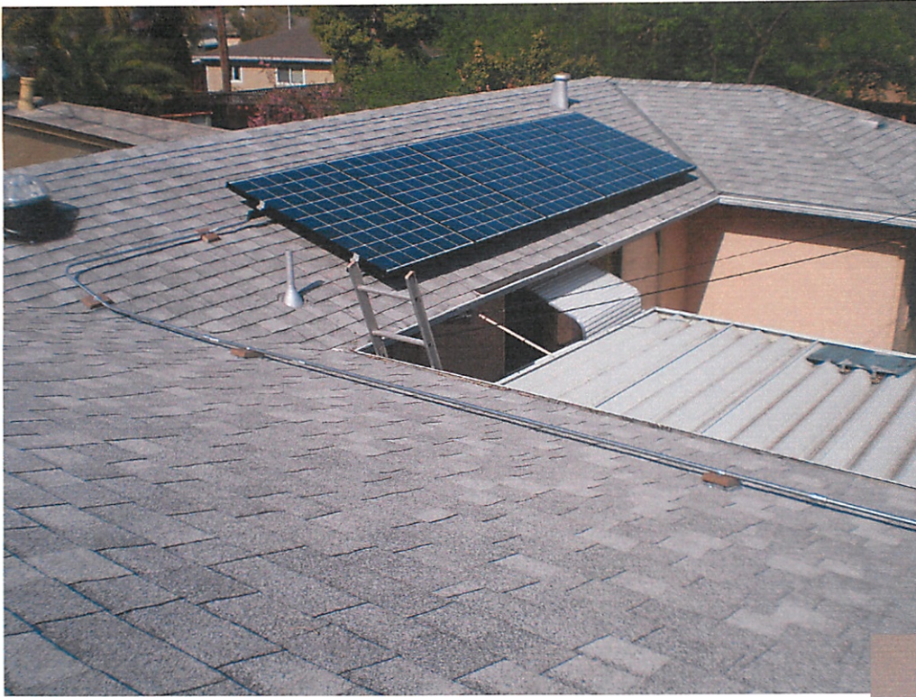
Five Panels Over Sun Room
