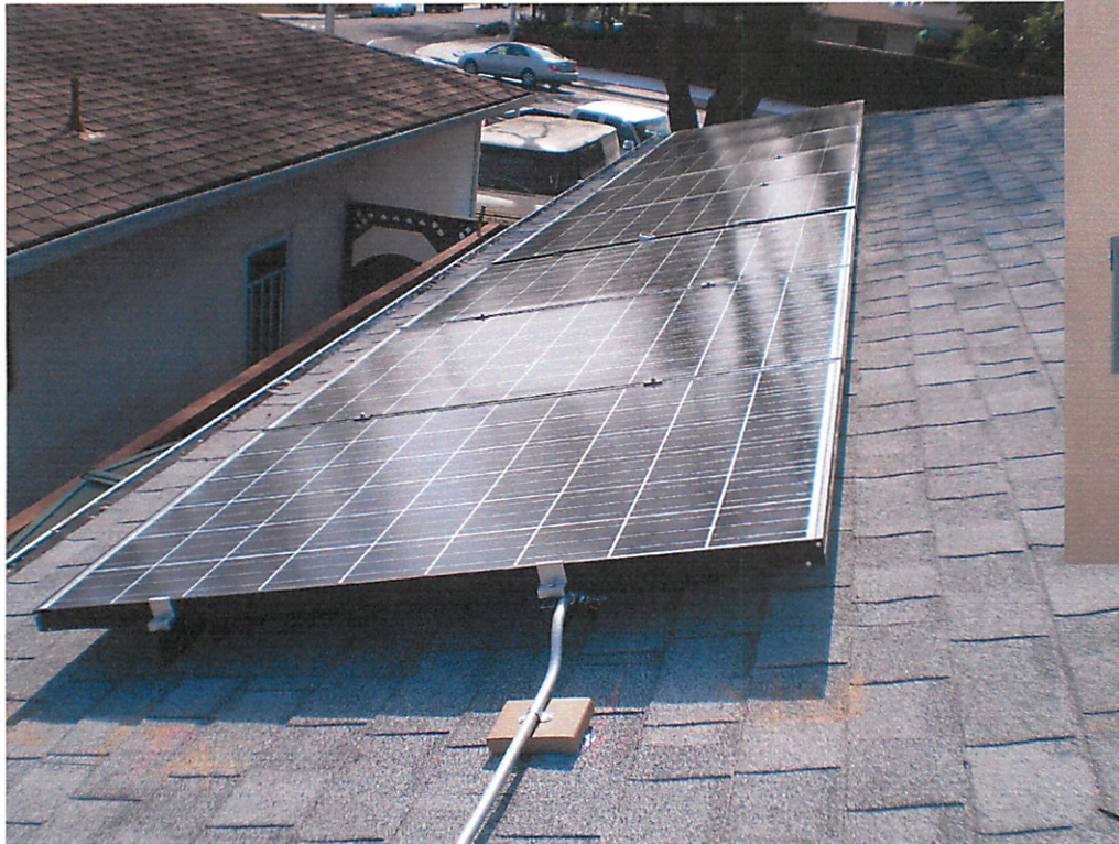
Eight Panels Over Garage
