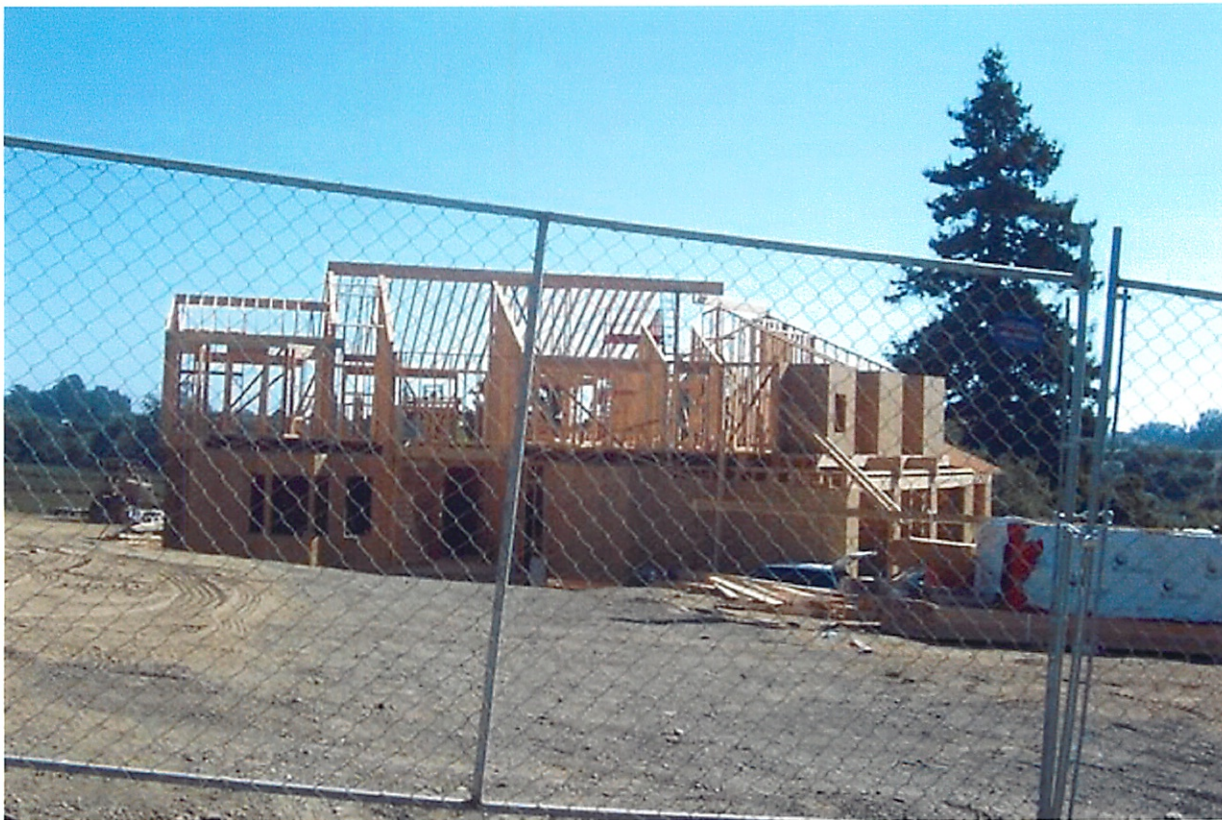
New Building on "Upper 60" of the old Green Valley Ranch 28 September 2008
