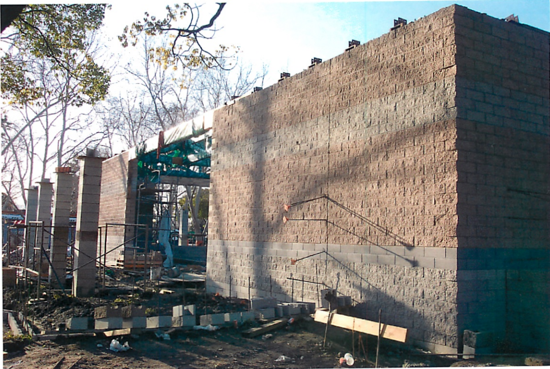
060109-001 Outside of new Senior Center swimming pool under construction.
