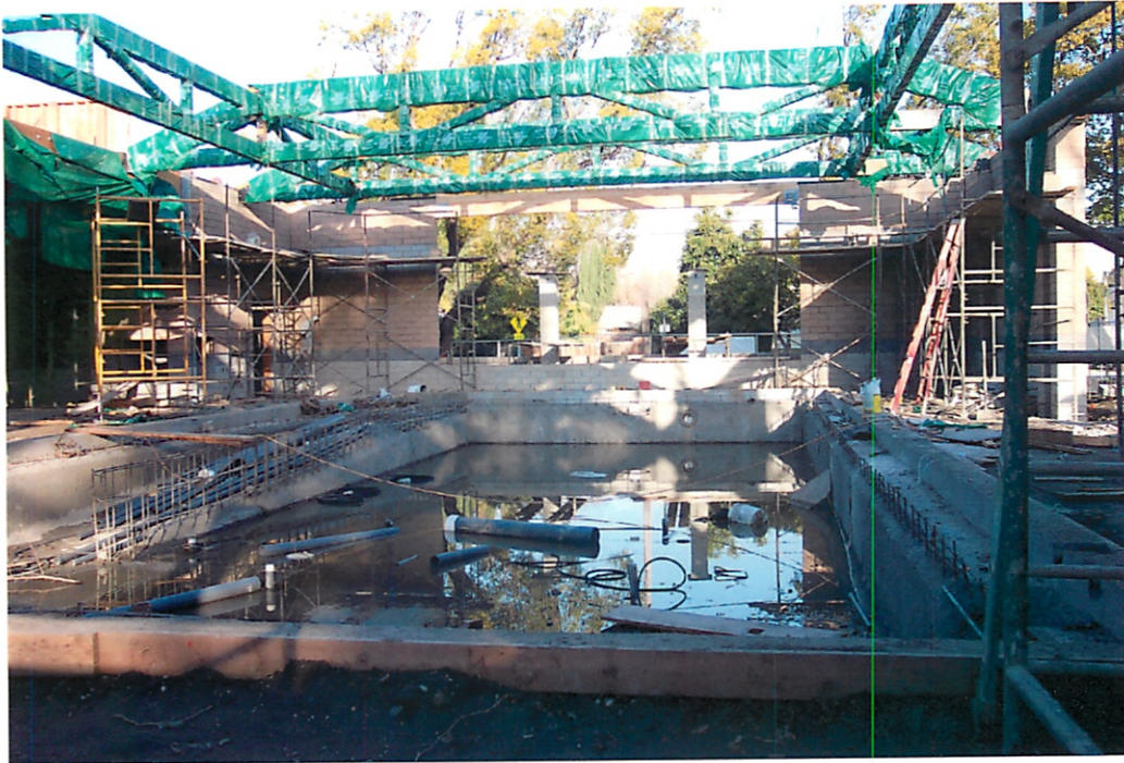
060109-002 Inside of new Senior Center swimming pool under construction.
