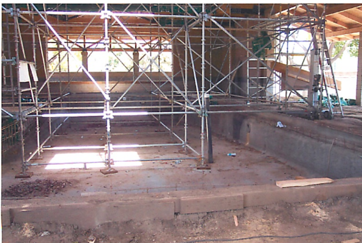
060511-036 New Senior Center swimming pool taken from west end looking east.
