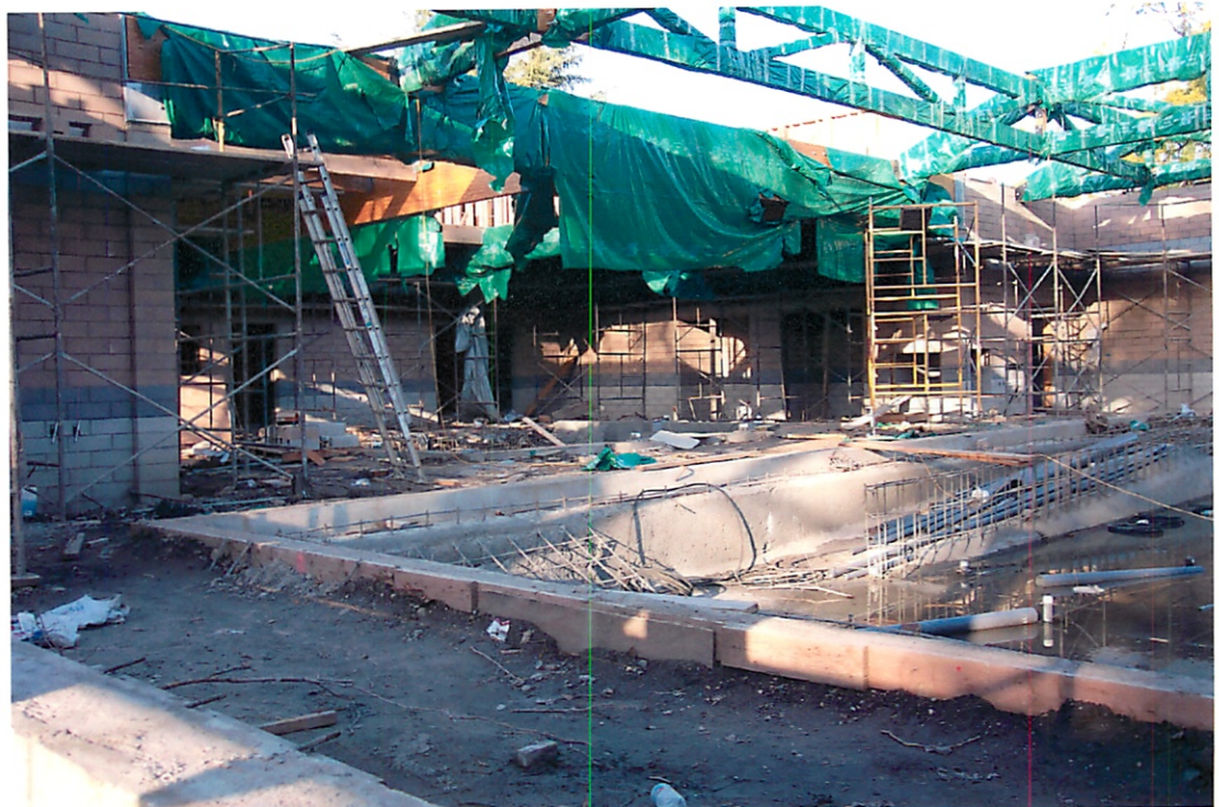
060109-003 Inside of new Senior Center swimming pool under construction.
