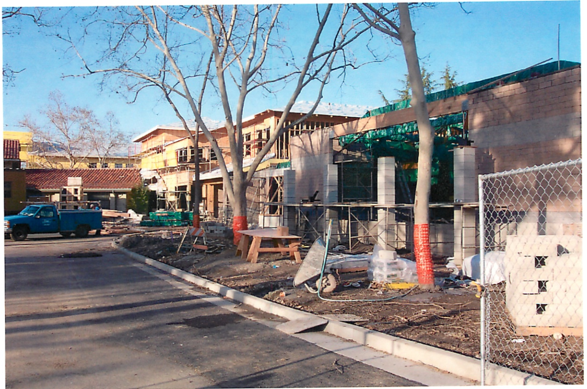
060109-004 Front facing driveway of new Senior Center swimming pool under construction.
