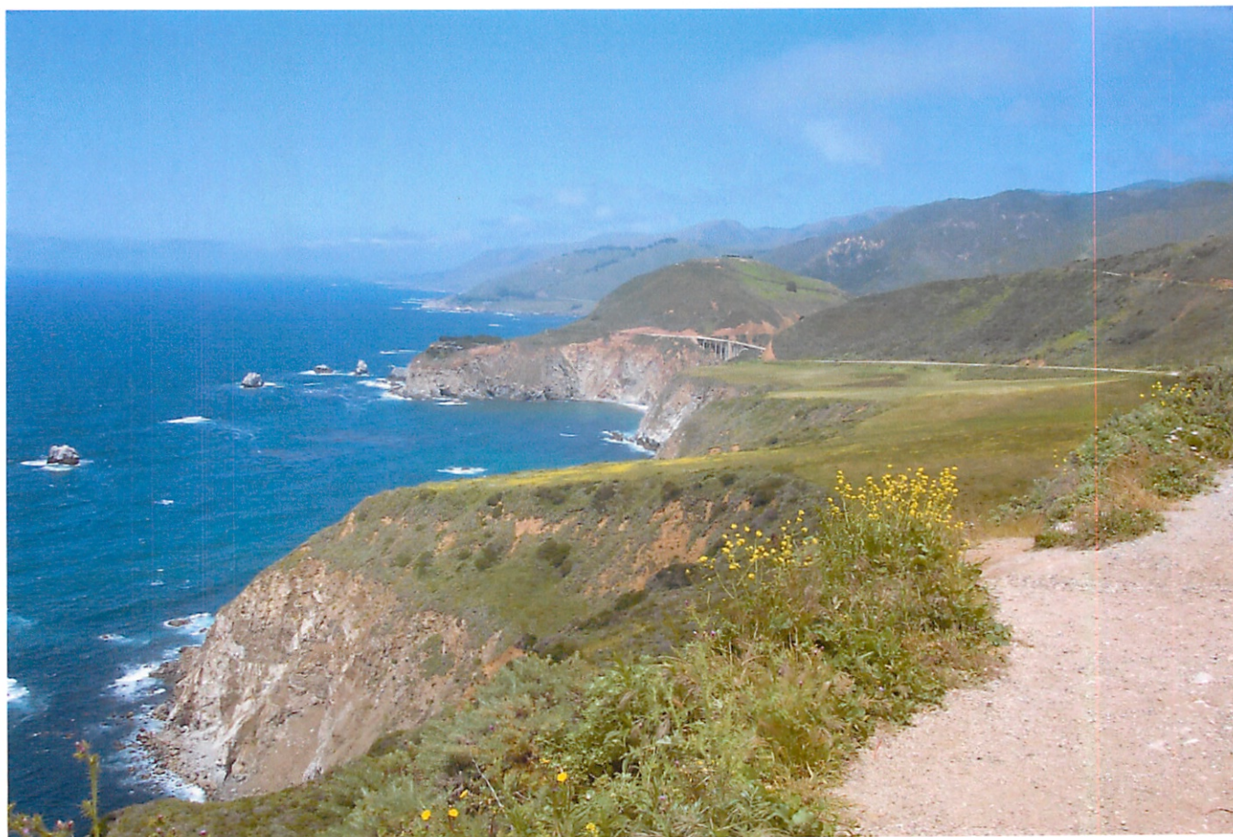
050511-049 Looking north at Bixby Bridge from Coast Highway (Highway 1).
