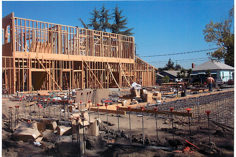
050928-163 Construction of addition to Santa Clara Senior Center.
