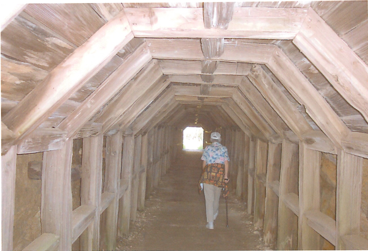
050513-087 Janet inside tunnel at Partington Cove.
