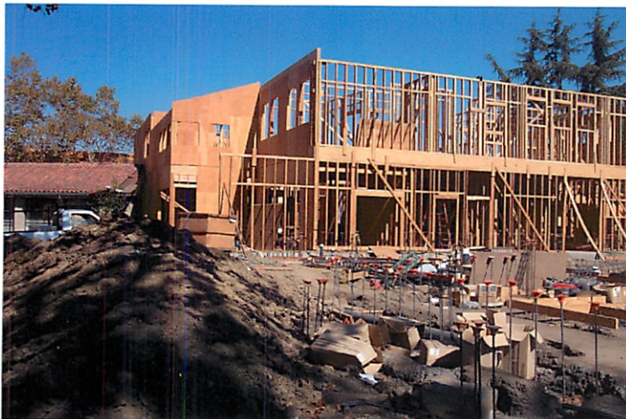
050928-164 Construction of addition to Santa Clara Senior Center.
