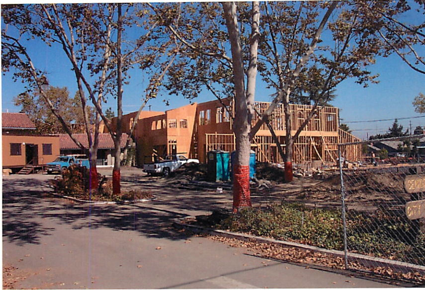
050928-165 Construction of addition to Santa Clara Senior Center.
