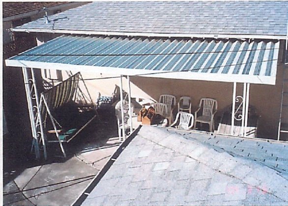
04-01-06 Patio and patio cover taken from roof of our house at 631 Kiely. 13 March 2004
