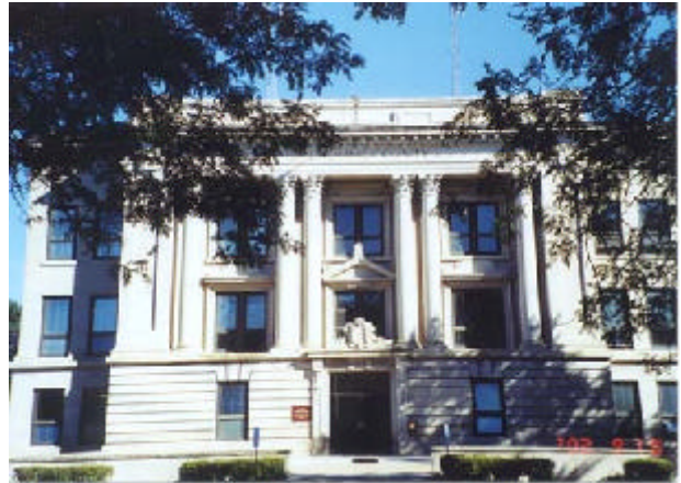
Bon Homme County Courthouse 16 September 2002
